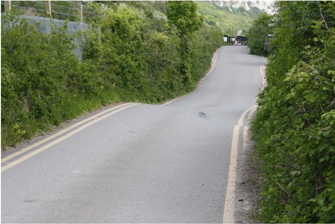
Figure 30 Road by railway flexed over an old slip.
