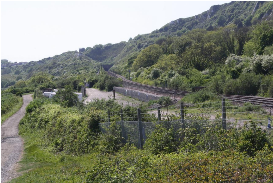
Figure 31 Gabions supporting the kink in the railway line.
