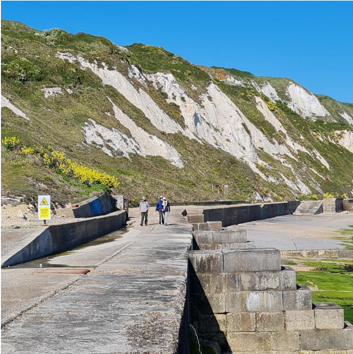
Figure 28 Concrete bench on the foreshore at Folkestone Warren designed to load the toe of the slips.
