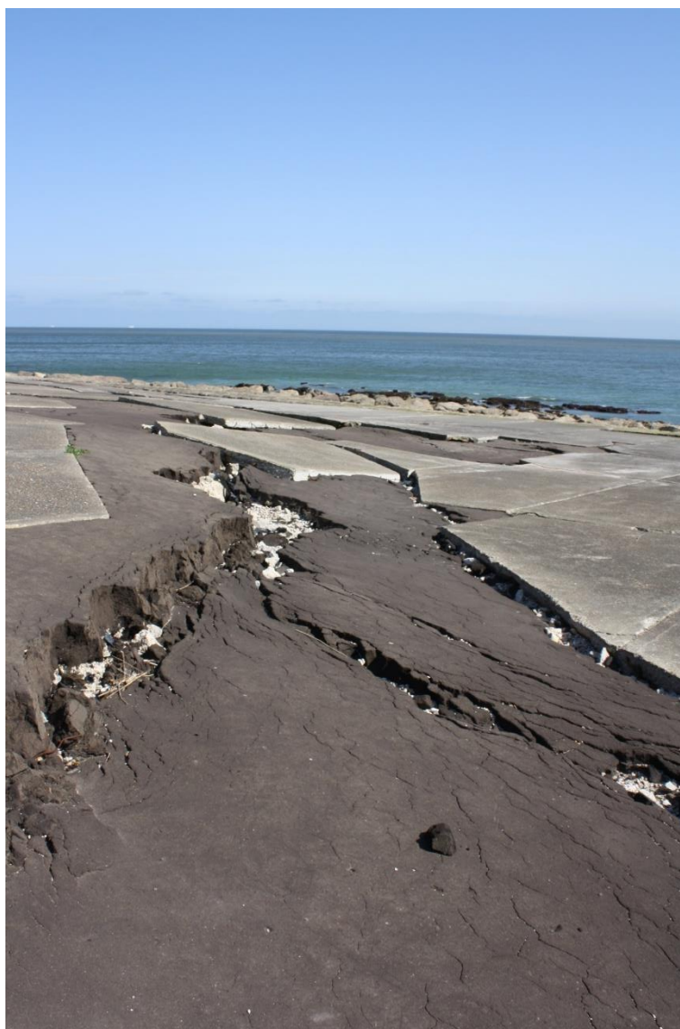
Figure 34 Displaced concrete slabs and asphalt caused by erosion of the toes of the slides
