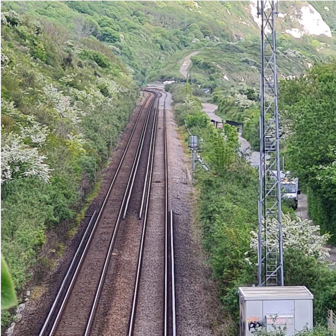
Figure 24 Kink in the Folkestone to Dover railway caused by previous land slips.
