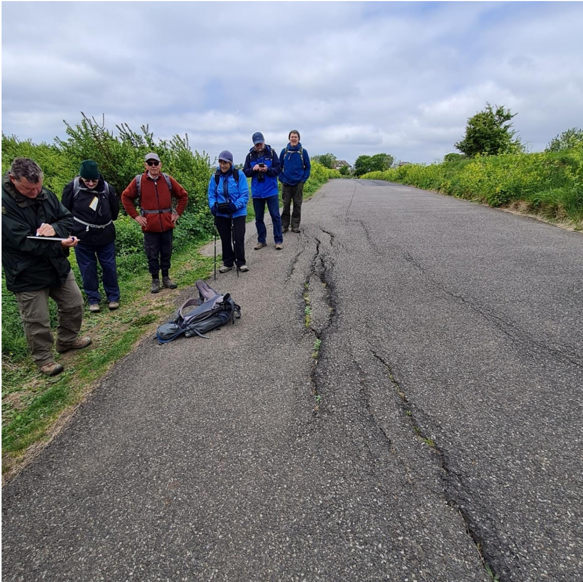
Figure 25 Cambering and fracturing of the Old Dover Road at Chapel-le-Ferne.
