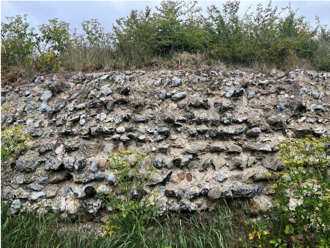
Figure 14 Core material in the southern wall of the Roman fort at Reculver.
